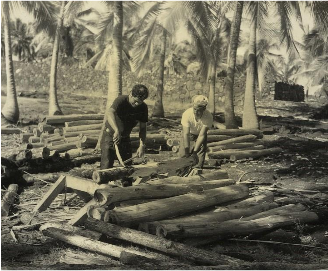
Figure 12. . Restoration: (Left to right) James Simmons and Clarence Medeiros, Sr. shaping palings to surround Hale o Keawe. (Photograph by Russell Apple, 1966; Negative No. 1797. Courtesy of National Park Service, Pu‘uhonua o Hōnaunau National Historical Park; Collection Number; PUHO 5461 series IV; Images; Boxes 50-54)
