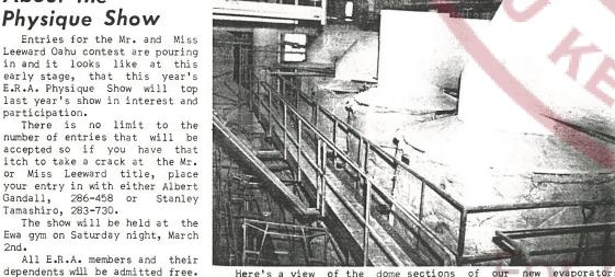
Here's a view of the dome sections of our new evaporators where the Associated Insulation Company is continuing their work insulating all cells and vapor pipes. Work on this project is estimated to be 50 per cent complete.
