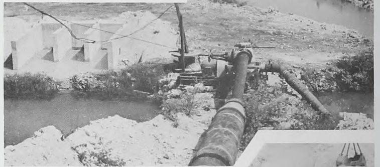
WORK IN PROGRESS ON PUMP SITE NEXT TO FIELD 90.
