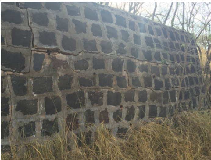
The retaining wall at Honouliuli predates the camp
