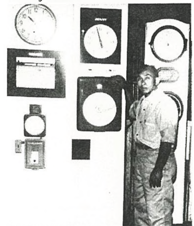
Sabas Bacon shows you the recording instrument mounted on the fireroom instrument panel.
