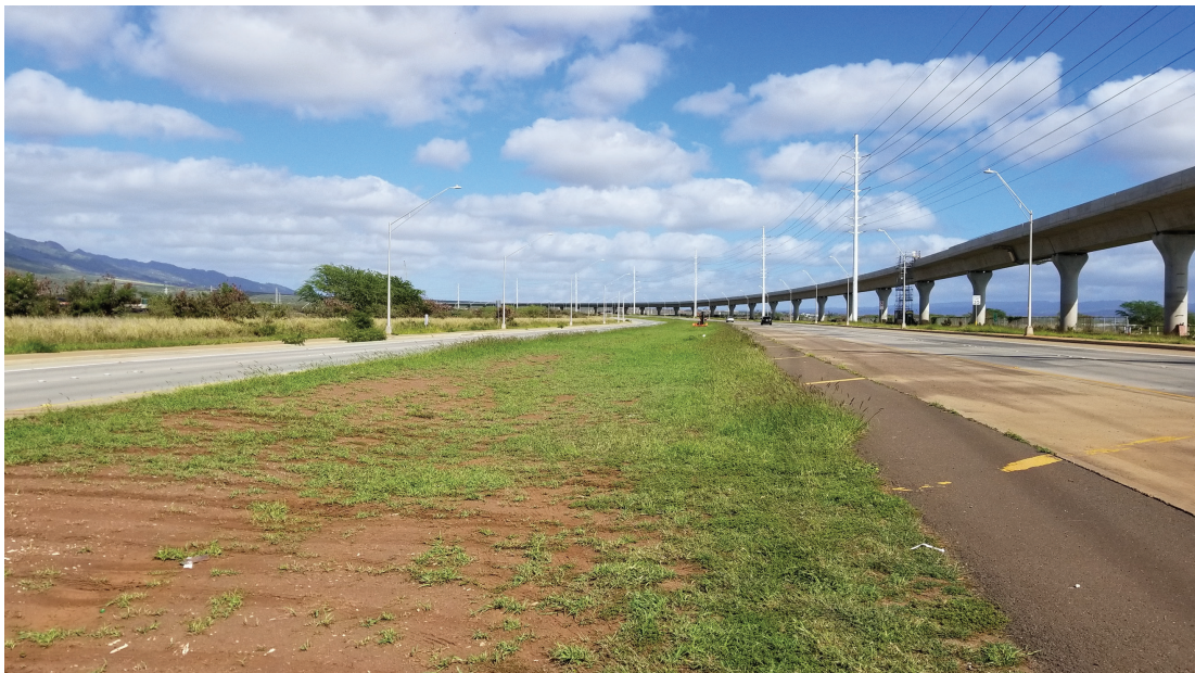
Fig. 1. Section view of a bioswale in practice along Kualakai Parkway road in Kapolei, Oahu, Hawaii.
