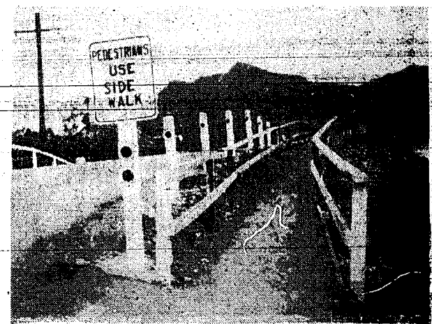
WHEN A MAN tired of stalling at city hall threatened to build this road and walkway with 25 mothers to replace a muddy, dangerous mound, city hall made a contractor put in the roadway and path seen above. (See Story Page 7)
