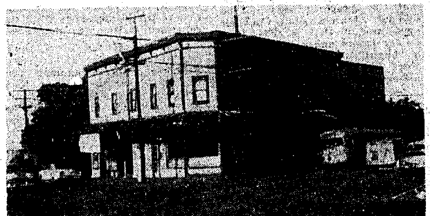
THIS BUILDING at the corner of Beretania and Alapai Sts. will disappear if and when the city buys the five acres it earmarked for a new police station.
